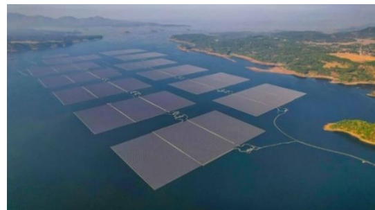
Figure 3 Cirata Floating Solar Power Plant (PV)
