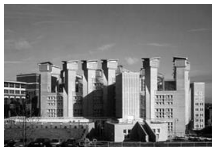
Figure 3 Actual application of stack ventilation towers at The De Montfort University, UK (above), and Frederick Lanchester Library, UK (below) [7]
