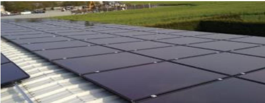
**Gambar 5. Solar cell Cadmium telluride (CdTe)**
