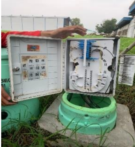
Gambar 1. Optical distribution point (ODP)
