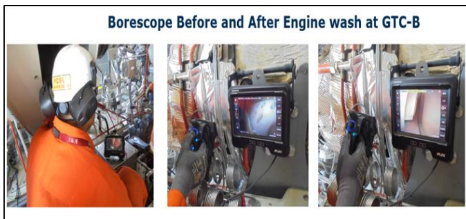
After Engine Wash at GTC-B
